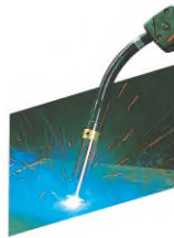
CO 2 /MAG Welding
